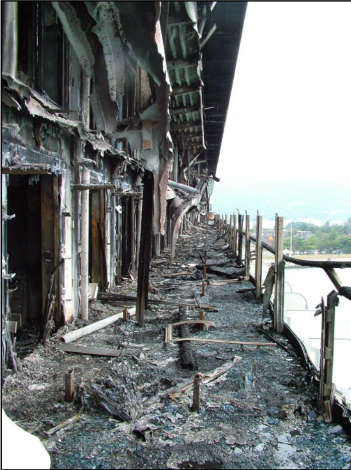
Melted aluminium structure
