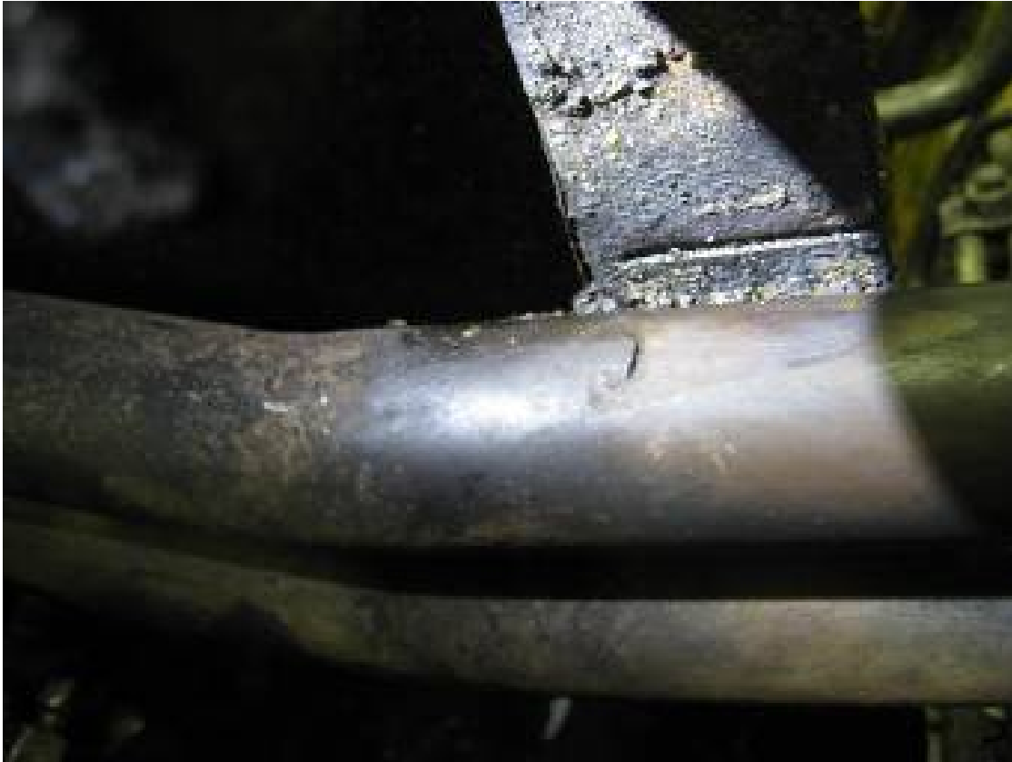
View of the fuel line split at the point where the line enters the hot box at the aft (turbo charger) end of engine No. 4
