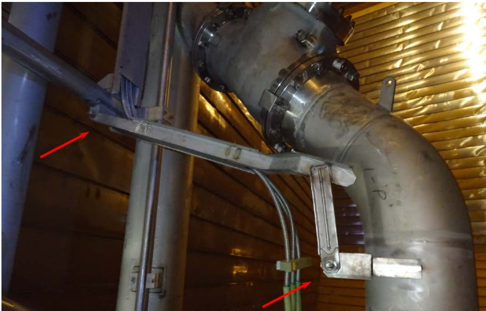
Fig. 2: Cable tray following repair
